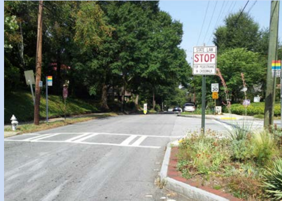
Marked and Signed Crossing to Transit Stop (Atlanta, GA)
